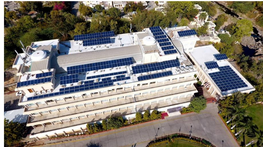
HZL's corporate office - Yashad Bhawan is Rajasthan's First CII-IGBC Certified Platinum Green Building
