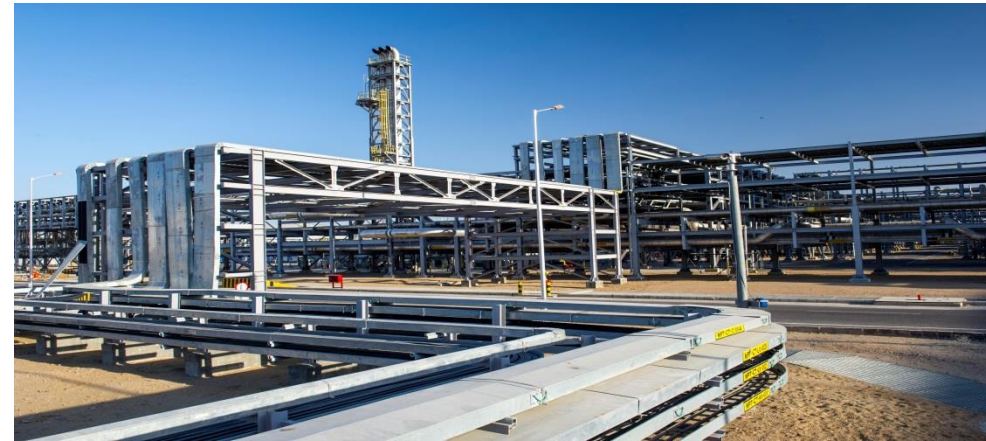
Rajasthan: Mangala Processing Terminal
