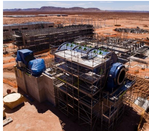
Erection of Ball Mill Shells, Bearing Housing & Motor
