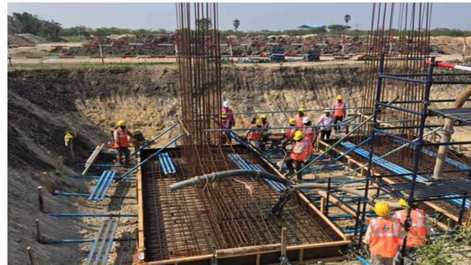
Construction of Tuticorin II (400kt)
