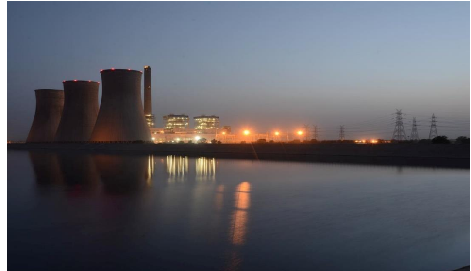
Talwandi Sabo Power Plant
