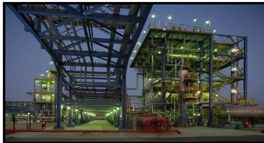
Rajasthan: Raageshwari Gas Terminal
