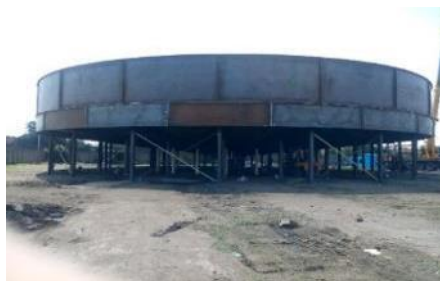
Thickener pre-assembly test
