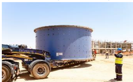
Mill shell on site
