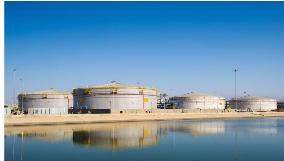
Rajasthan: Mangala Processing Terminal
