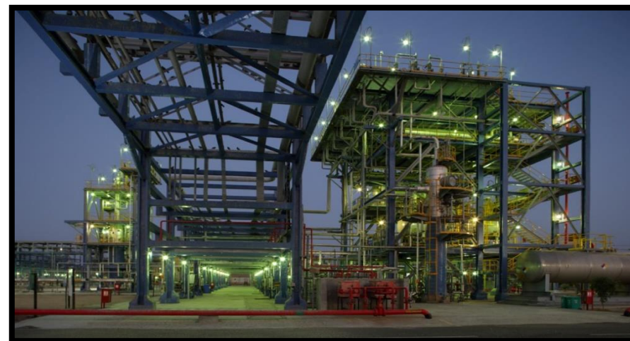
Rajasthan: Raageshwari Gas Terminal
