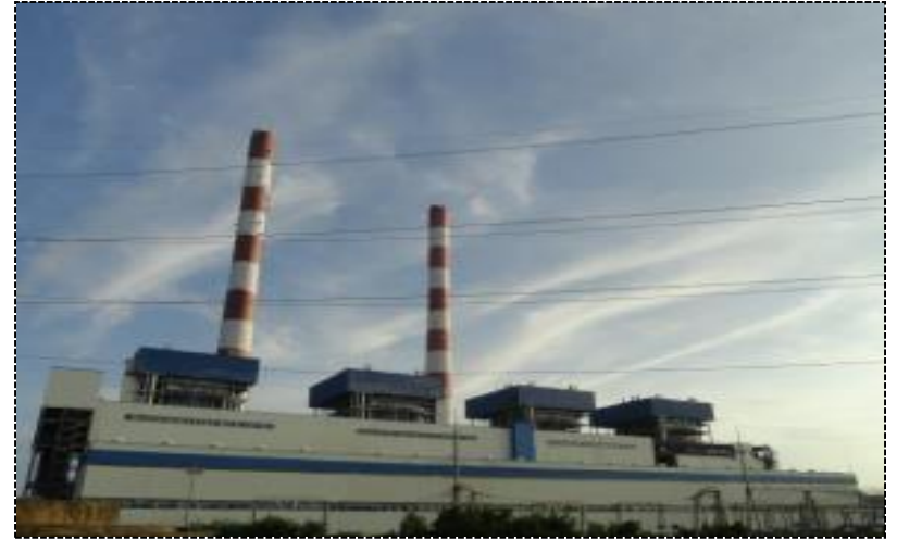
CPP 540 MW in smelter Site
