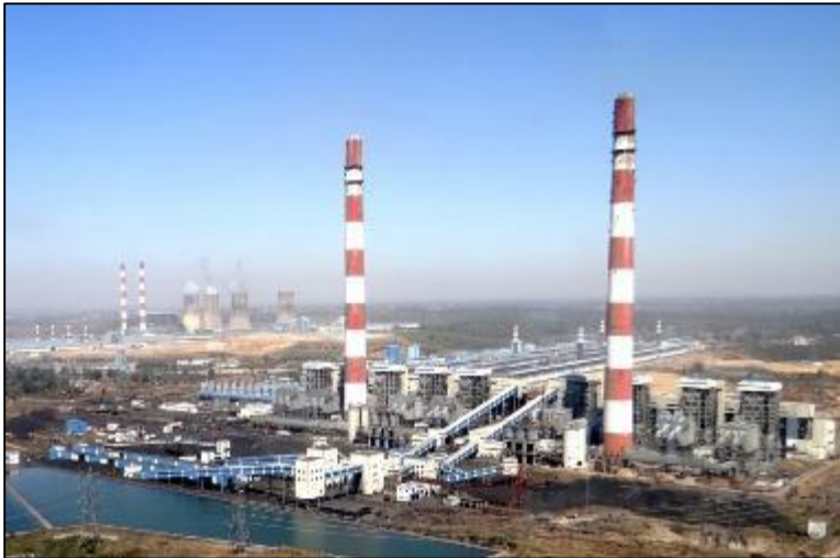
1215 MW Captive Power Plant
