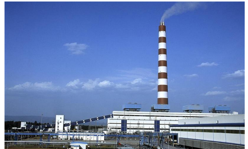
CPP 1200 MW in smelter Site
