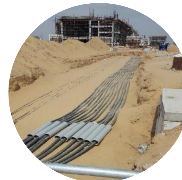
Cable Laying- Compressors
