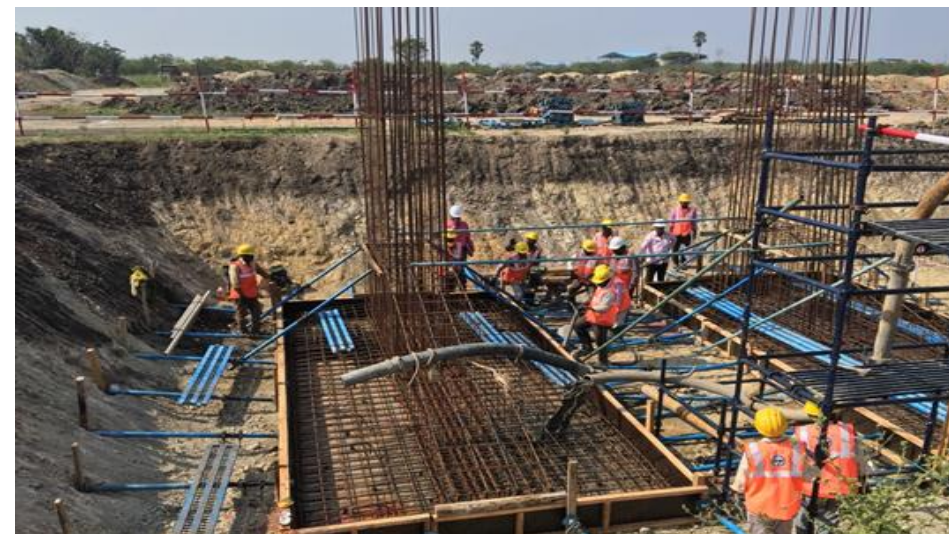
Construction of Tuticorin II (400kt)
