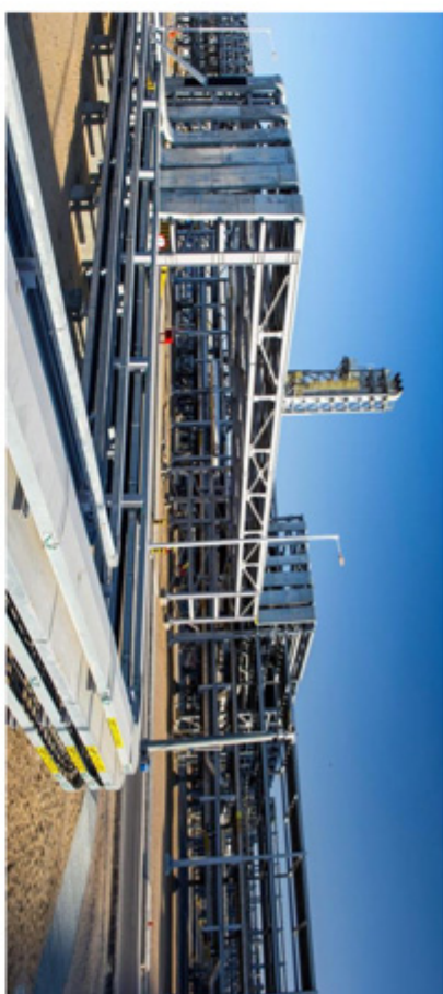
Rajasthan: Mangala Processing Terminal
