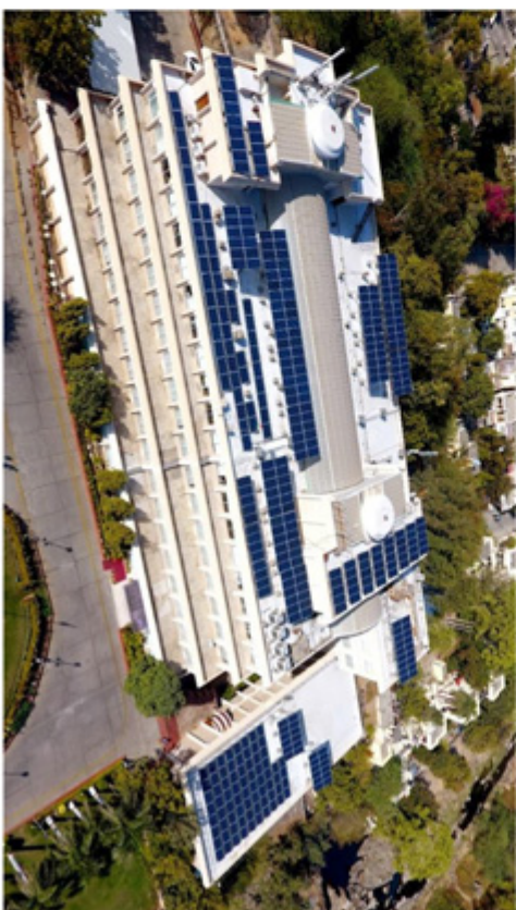
HZL's corporate office - Yashad Bhawan is Rajasthan's First CII-IGBC Certified Platinum Green Building
