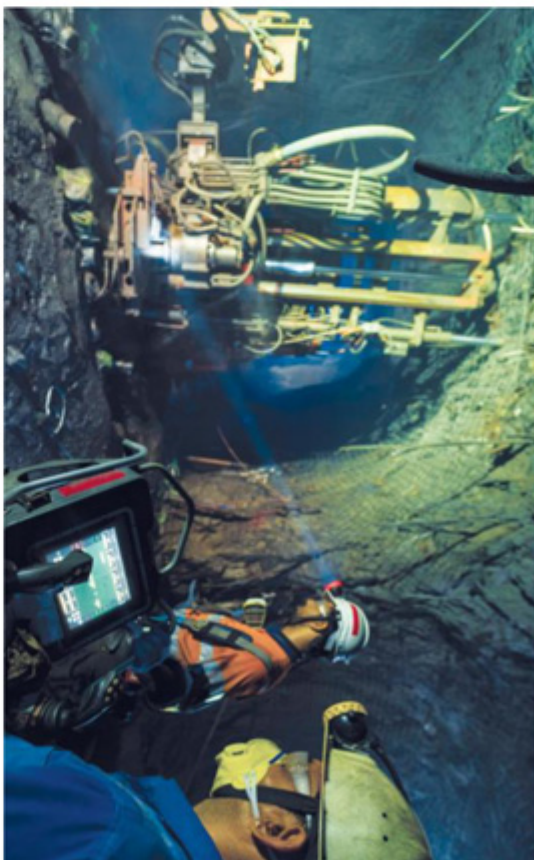
Long-haul drilling machine at work
