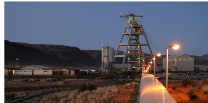
Deeps Shaft, Black Mountain Mine, Aggeneys
