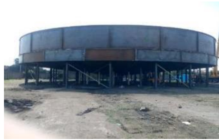
Thickener pre-assembly test
