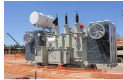
Transformer installed on site
