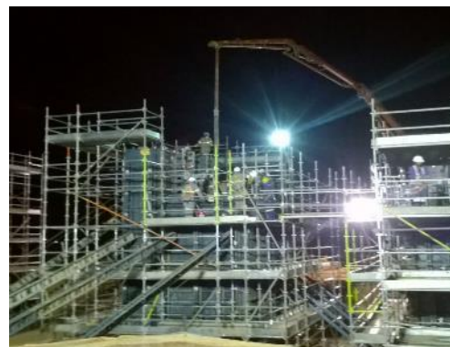
Ball mill foundation
