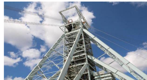
Konkola deep mine shaft
