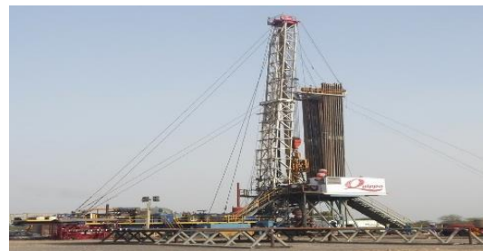
Well Spud at RDG in April 2018
