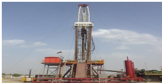
Well Spud at Aishwariya EOR in April 2018
