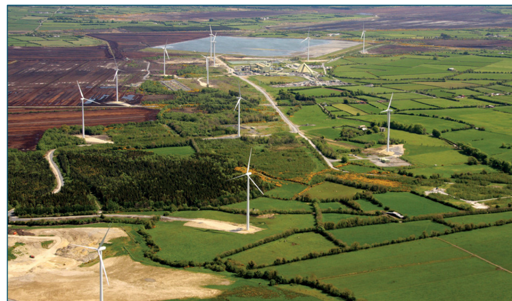
Lisheen Windfarm Project
