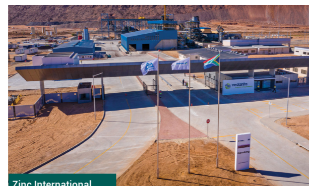
Zinc International Gamsberg Plant
