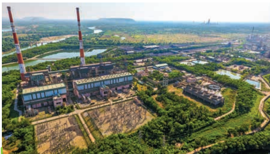
Below: Captive Power Plant at Chanderiya Smelting Complex
