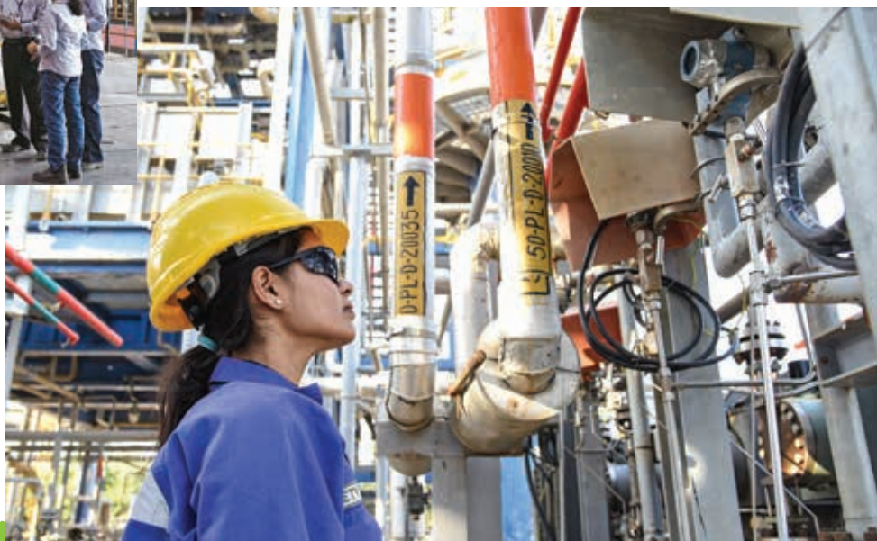
Right: Employee at operational site, Cairn Oil & Gas
