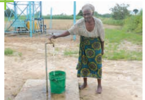
Above: Chingola peri-urban solar powered borehole: Harvesting the sunlight
