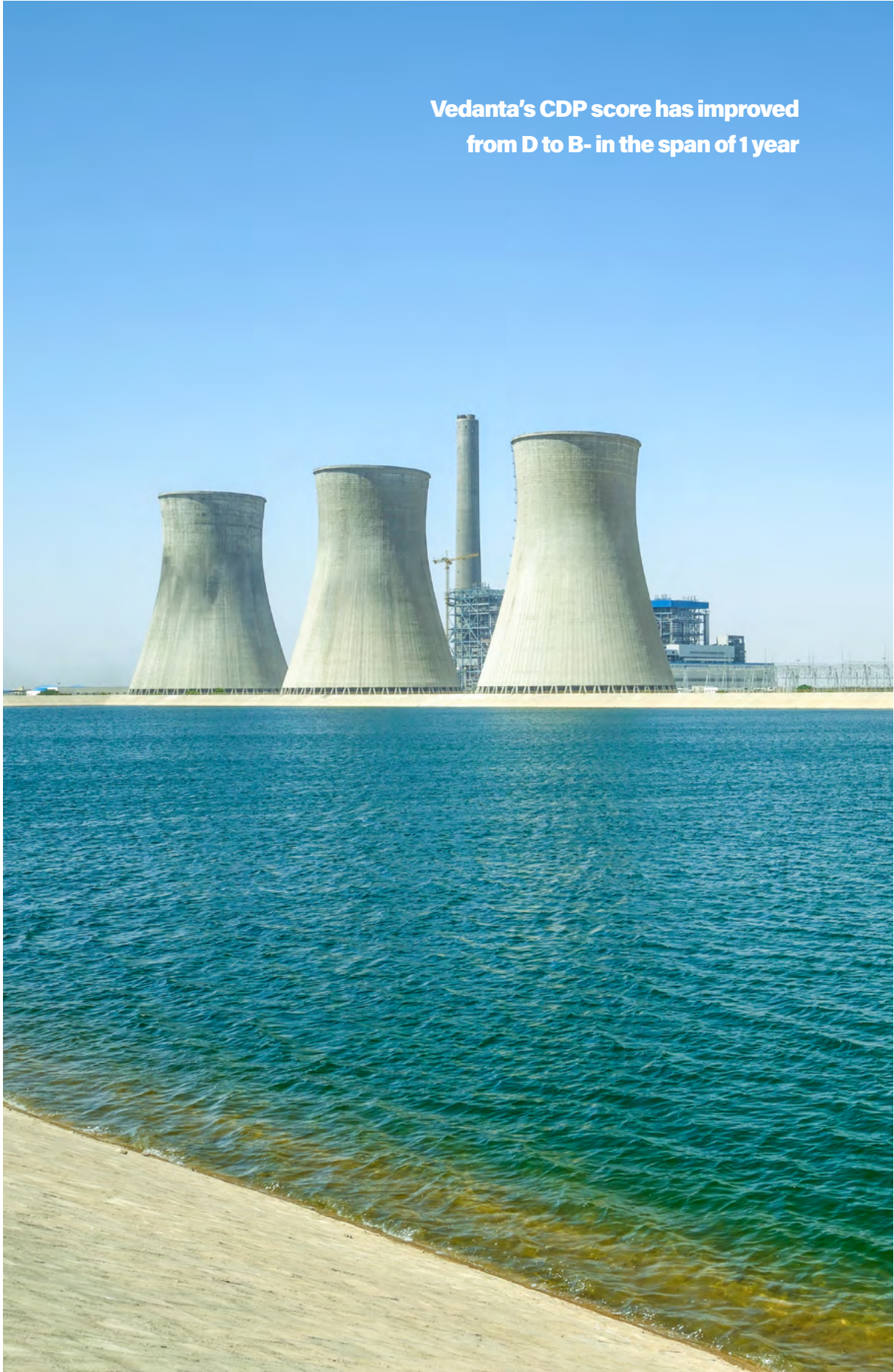
Power infrastructure at TSPL
