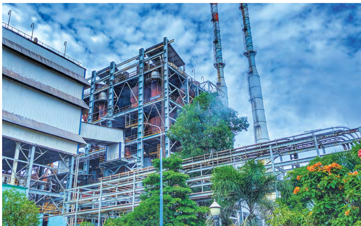
Calciner plant in Lanjigarh alumina refinery
