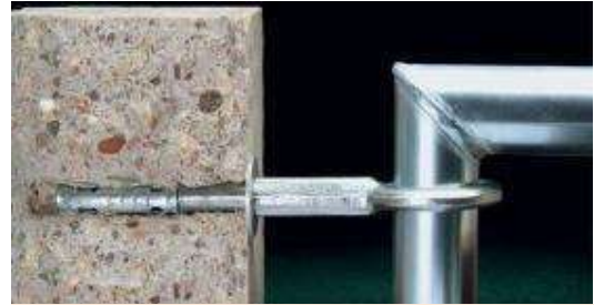
Figure 19: Tying the Scaffold to the Wall using a drilled in anchor
