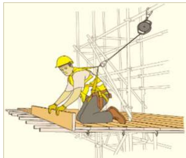
Figure 94: Falling object protection fan erected using an inertia reel
