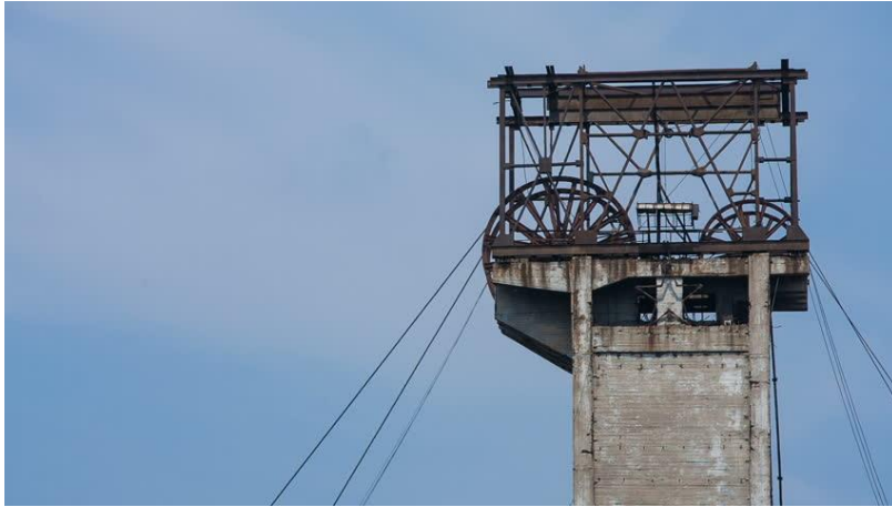
Winder Drum Management of water reticulation systems
