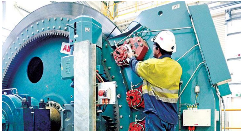
Mine hoist maintenance
