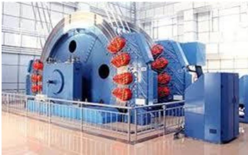
Mine hoist system
