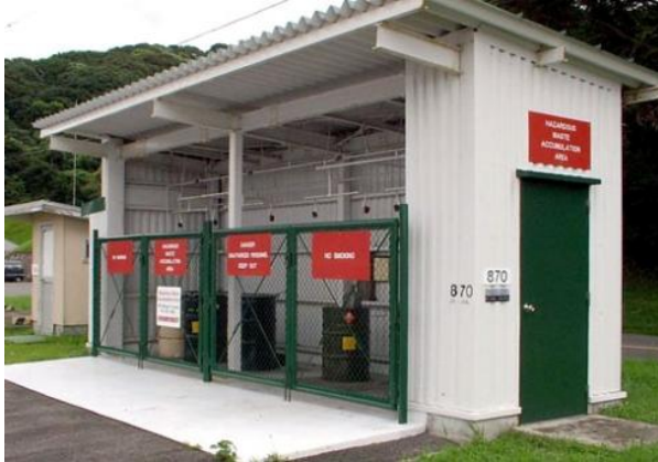
A typical secure, sheltered, waste storage area
