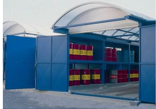
A typical dedicated storage area for multiple waste types
